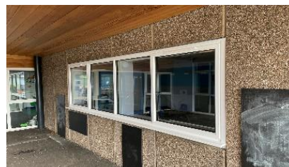
Kingsway Primary School
