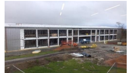
The Telford Langley School new classrooms building
